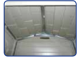
Galvanized Steel Roof Trusses and Wall Support
