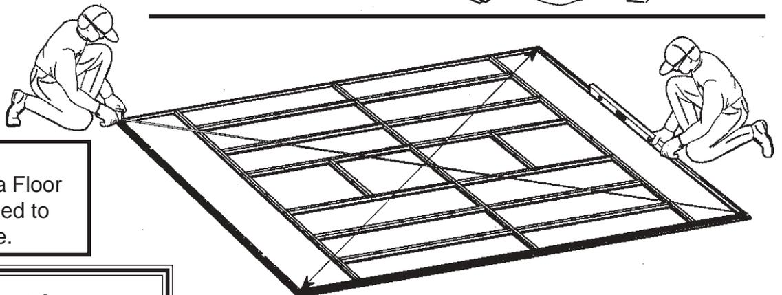
**The floor frame *must be square and level* or holes will not align.**
